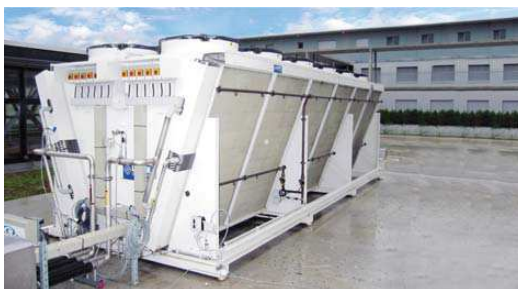
Rys. 9. CO 2 gas-cooler z systemem zraszania
