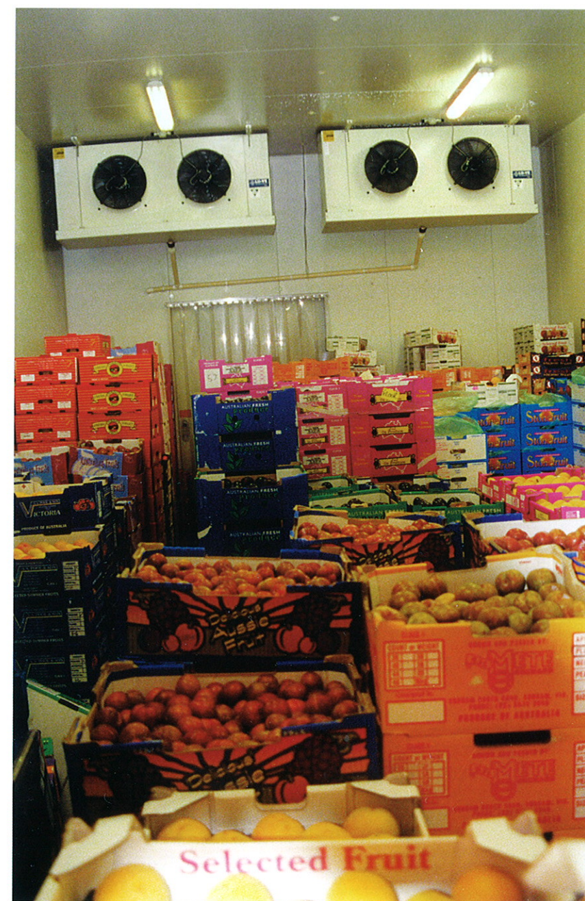
Two LU-VE Evaporators NHI 587 N 3 with 25k W capacity
